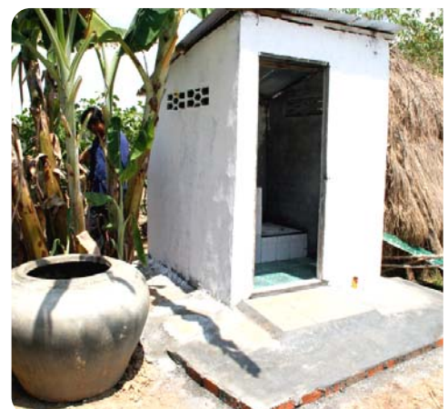
Corporate funding enables toilet construction in rural Maharashtra
